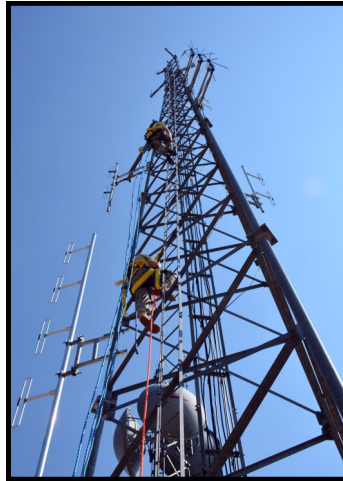
120th CF members Tech. Sgt. Michael Hedrick and Tech. Sgt. Josh Petersen climb a 100 foot communication tower. U.S. Air National Guard photo/Senior Master Sgt. Eric Peterson)
