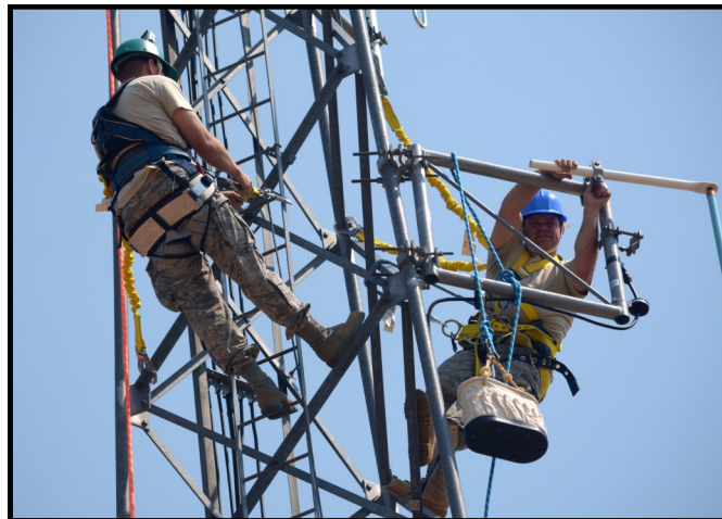
120th Communications Flight members Tech. Sgt. Michael Hedrick and Tech. Sgt. Josh Petersen install antennas on a communication tower. U.S. Air National Guard photo/Senior Master Sgt. Eric Peterson)
