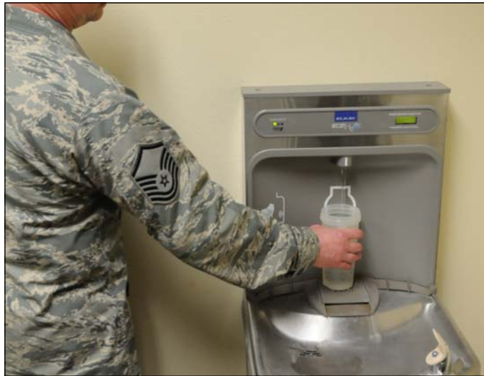
An Airman fills his water bottle from a water fountain that filters drinking water. The filter is not needed to make the water safe to drink, but makes it taste better. National Guard photo/Staff Sgt. Michael Touchette
